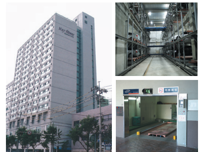
Cart parking (Multilevel dolly system / Pallet type)
