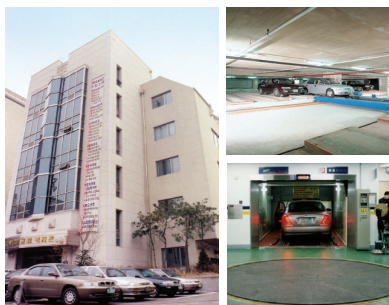
Trolley parking (Multilevel dolly system / No pallet type)
