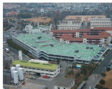
Free parking (Light-weighted and independent steel structure)
