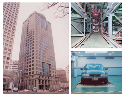
Shuttle parking (Multilevel dolly system / High speed type)
